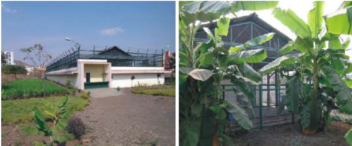
Enrichment of Infrastructure : Ecofriendly Monkey Enclosure, MCC, NIV, Pune.
